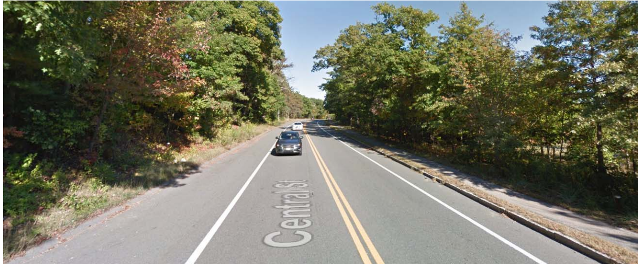
Exhibit 3 Route 135 Post-Road Diet (2016) – two-lanes along corridor with left-turn pockets
