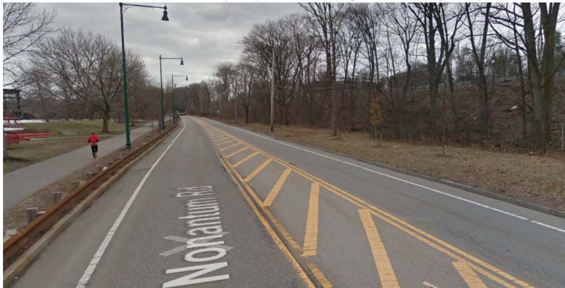
Exhibit 6 Nonantum Road Post-Road Diet (2016) – two lanes along corridor with left-turn pockets
